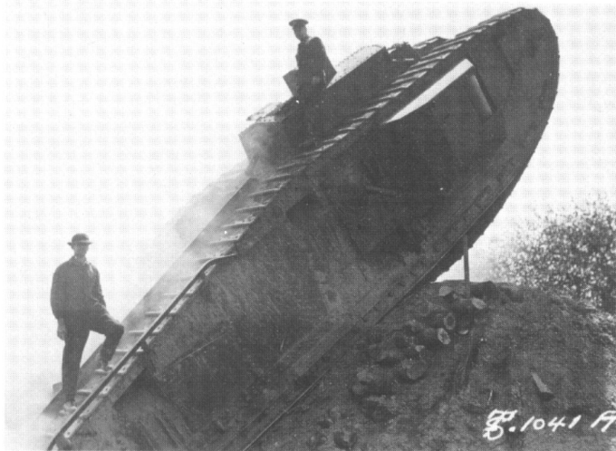
A Mark VIII being tested on a 39 degree incline at Aberdeen Proving Ground. Tank No. 67986 is producing a heavy amount of smoke created by a leaky oil system.
